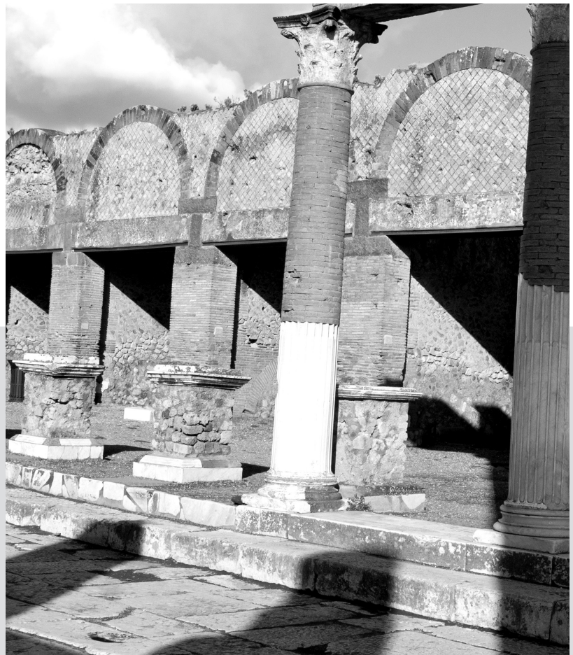
In the Forum of Pompeii, we can see another example of a builder using embedded arches to relieve the load on the lintels of a series of openings in the front of a building.
